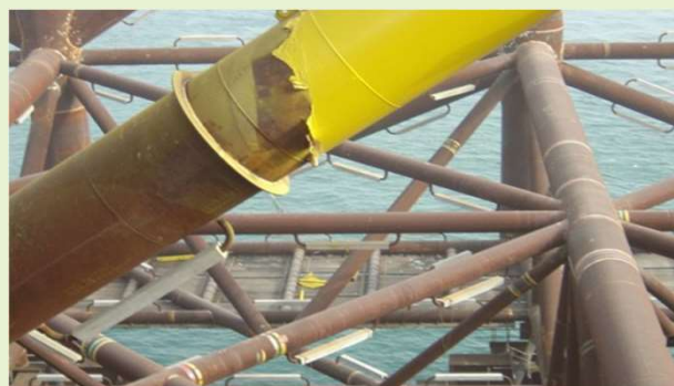
Jacket wind protection damages
