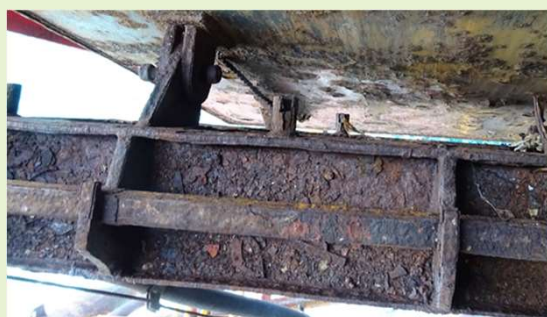
Corrosion of the pile of platforms
